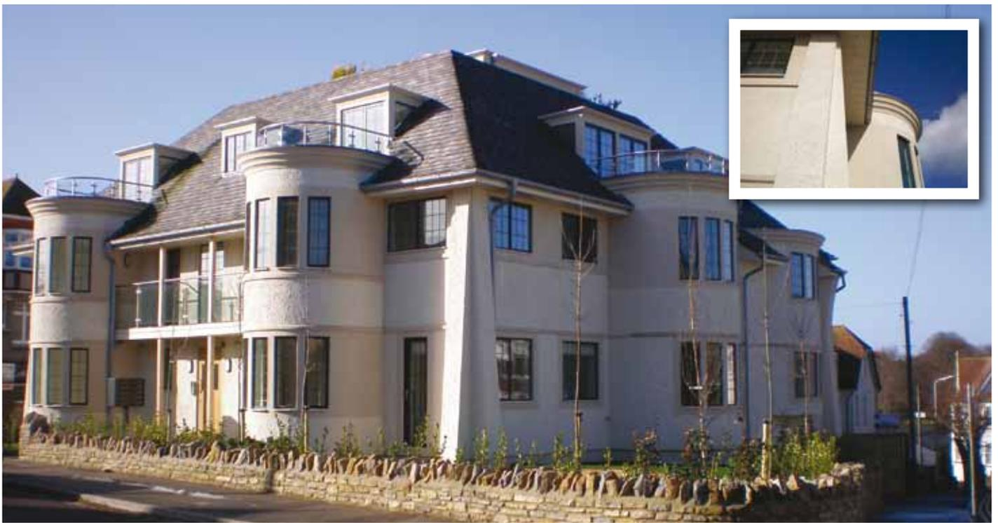
**S**wan Homes wanted to create a 1930s art deco building for their development of ten flats in the sea-side town of Swanage. The wall and roof structure is a timber framed modular package from Germany. Franco's task was to design and manufacture the three main components to the building comprising GRC curved cornices to the bay fronts, a pre-cast stone string-course to be set at the first floor level, and a heavy rough-cast, sprayed finish,
